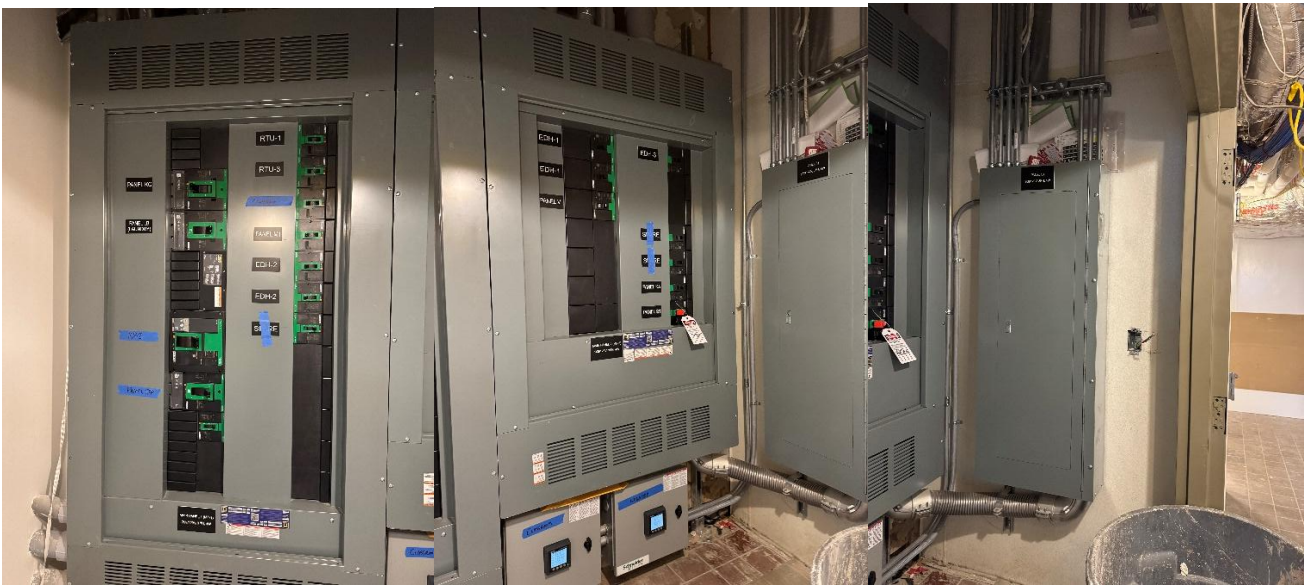
Figure 4: Elec 108 – Finalize Labeling, General Cleanup, Finalize Metering Connectivity, Light Switch
